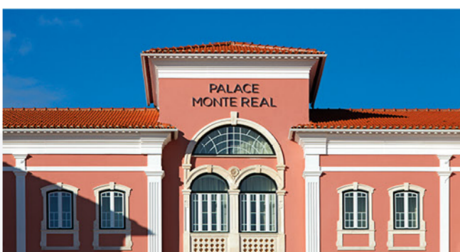
Palace Hotel Monte Real, Leiria António Garcia Arquitectos, Lda. Domus Natural Red
