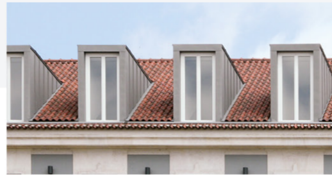
B Building, Praça D. Luis, Portugal Arq. Aires Mateus e Associados F3+ Rustic Natural
